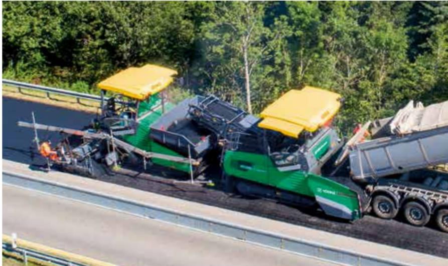
**T**he new **VÖGELE MT 3000-3 Standard** combines reliable technology with great operating convenience, making it even easier to transfer material to the paver without interruptions or jerks and thus ensuring top paving quality at maximum efficiency.
